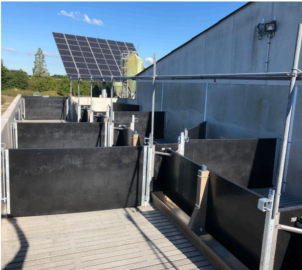
LOADING QUAY WITH RESIN TROUGH
